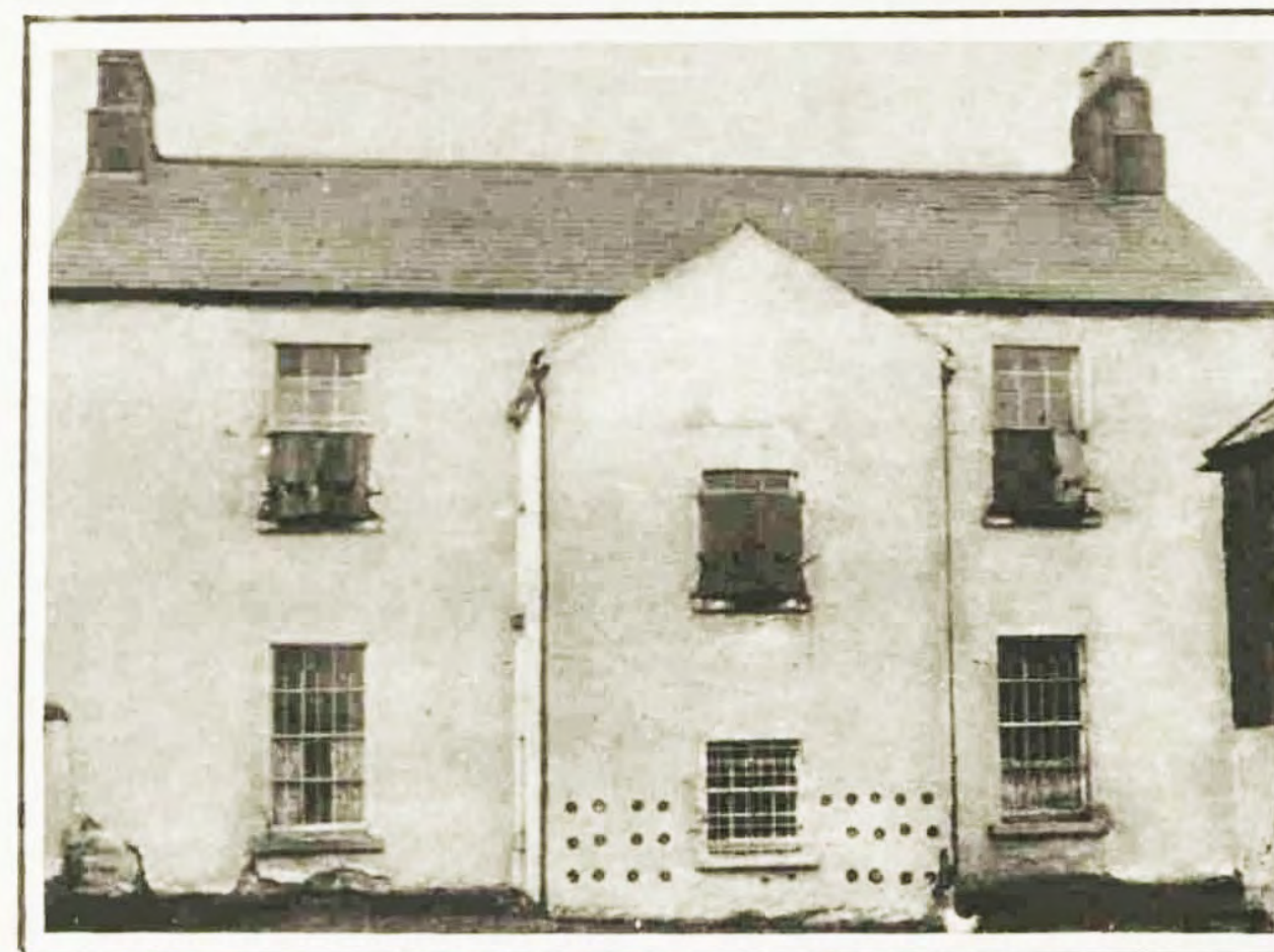
FORTIFIED WITH STEEL SHIELDS TO WINDOWS AND LOOPHOLES FOR RIFLE-FIRE: AN IRISH POLICE BARRACKS.
