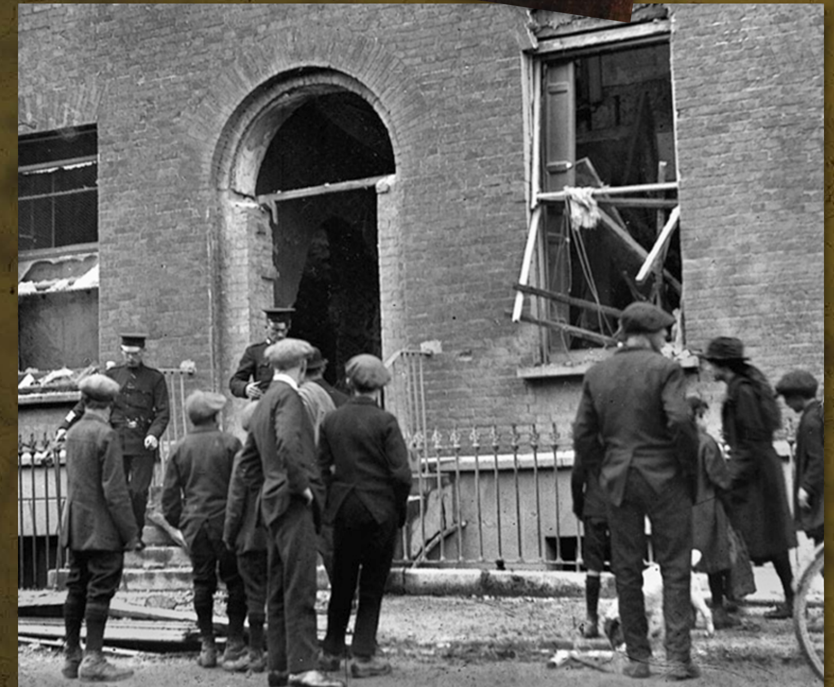
King Street (now MacCurtain Street) RIC barracks in Cork City after it was attacked and destroyed by Cork No.1 Brigade IRA on 20 July 1920 © Cork Public Museum Δ
