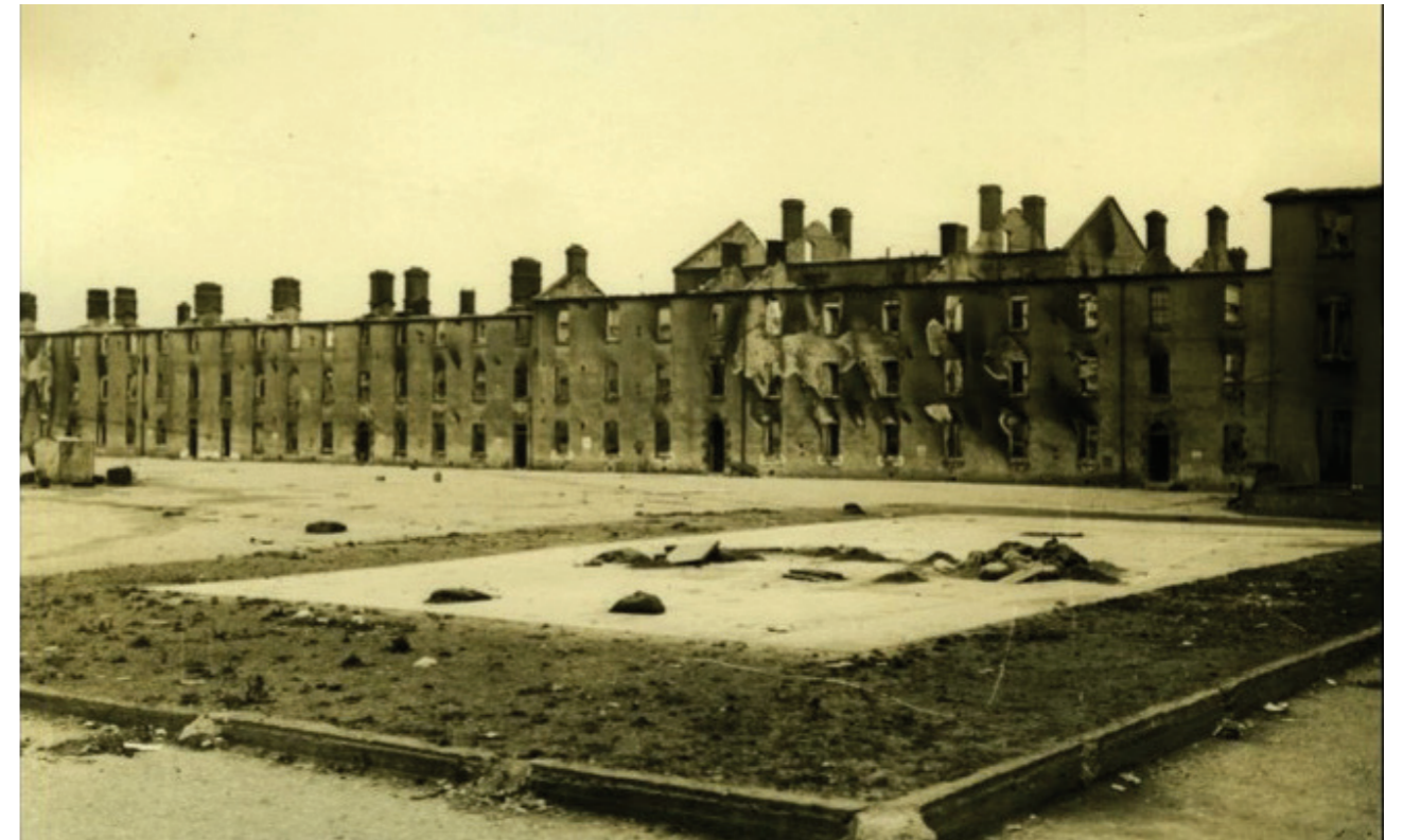
Fig. 31, Burnt out accommodation blocks at New Barracks, c. 22 July 1922
