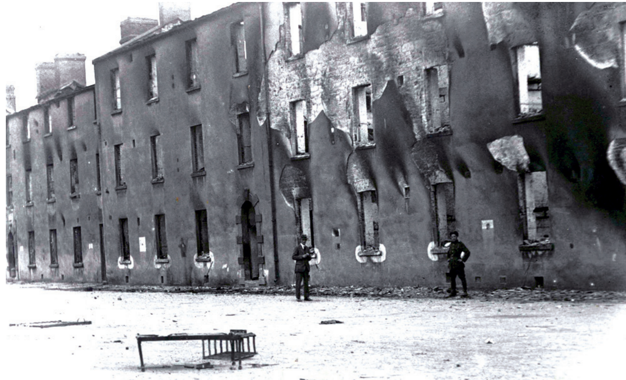
Fig. 30, Burnt out accommodation blocks at New Barracks, c. 22 July 1922
