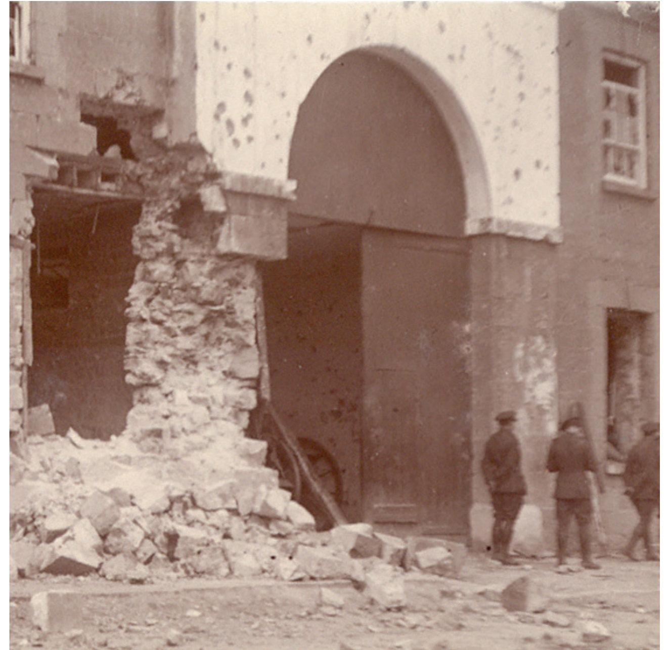
Fig. 52, National Army soldiers inspecting the ruins of Strand Barracks, c. 21 July 1922
